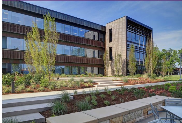
Figure 27 - Suburban Office Development Examples
